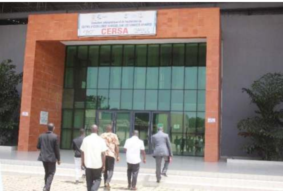
CERSA main building seen from the side and from the front
