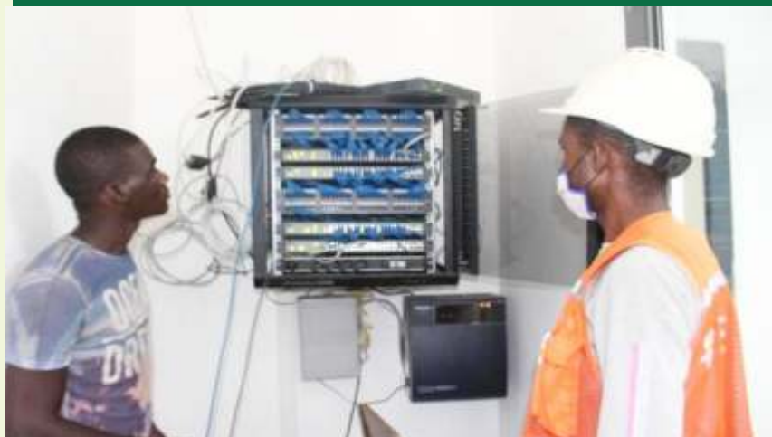
Telecom technicians during the installation of optical fiber at CERSA
